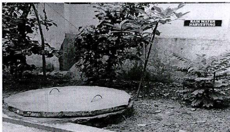
Fig.1: Rain Water Harvesting (RWH) system implemented in the College
